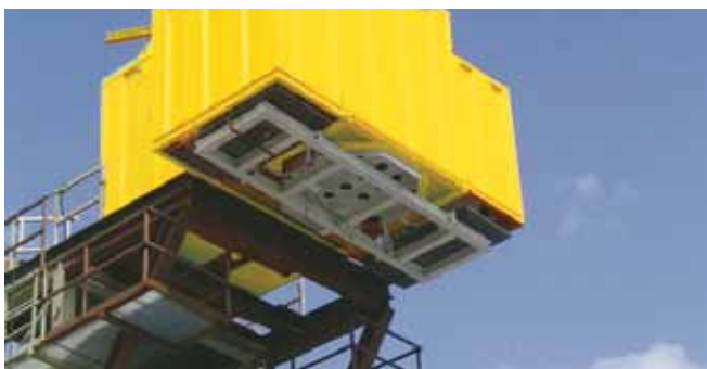
Container mounted at testing tower
